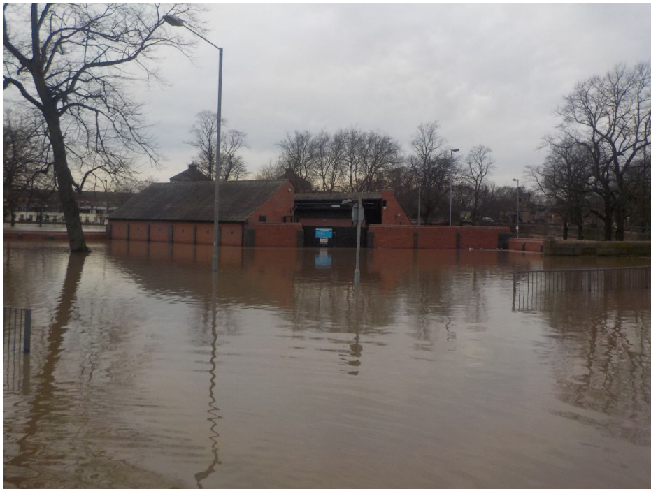
The pump-house compound
